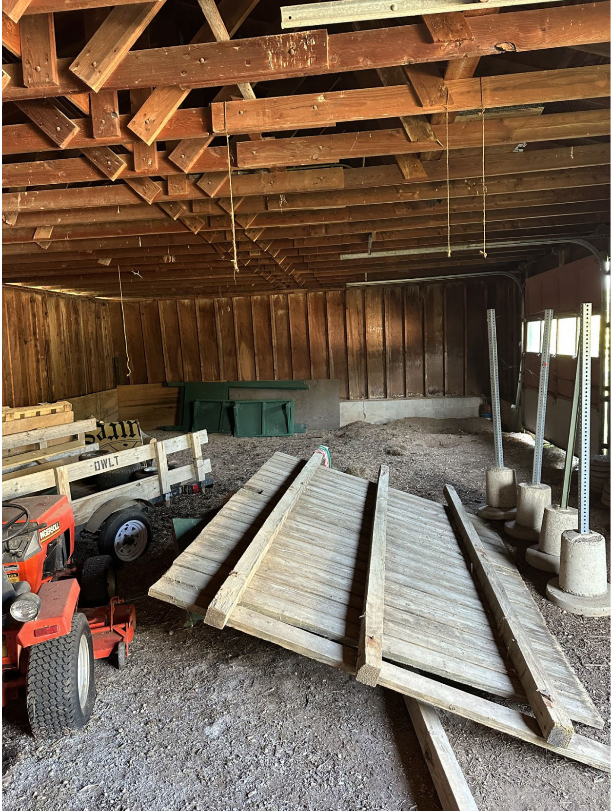
Dirt portion Storage Shed
