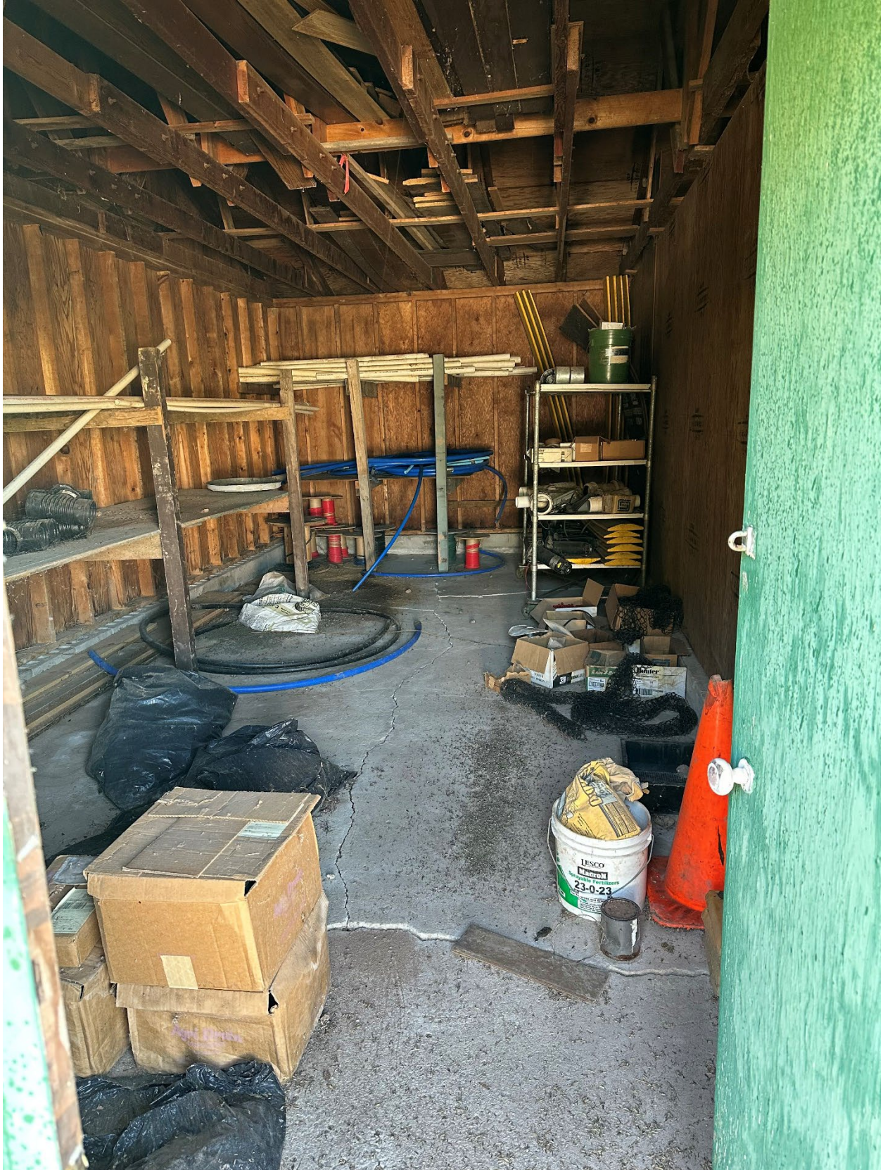
Concrete portion of Storage Shed
